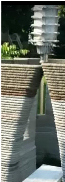
Figure 7: Cantilevered concrete layers additively extruded by TotalKustom. Source: TotalKustom.com
