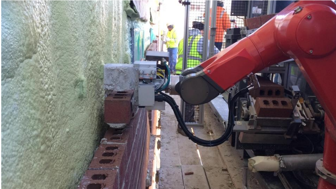
Figure 40: Semi-Automated Mason laying brick at Fort Lee Barracks in Virginia
