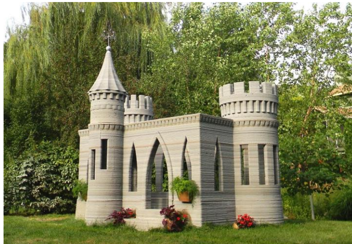
Figure 18: TotalKustom (Andrey Rudenko) 3D printed concrete castle
