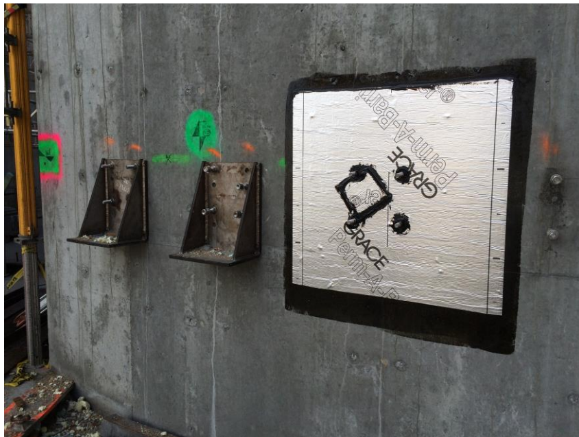
Figure 29: Bracket-anchor system to support Lecce Limestone Panels & waterproofing barrier on DRUM
