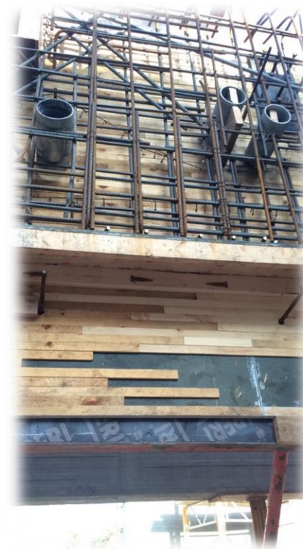
Wooden Board Forms in Steel Form
